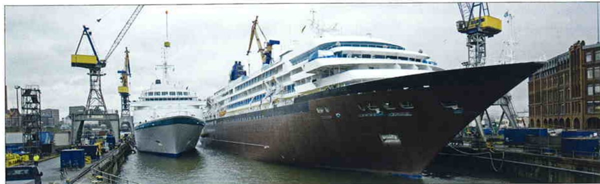
Booming repair and conversion, here at B+V Repair, is keenly contested
